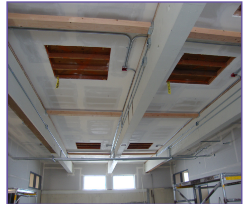
March—Skylight openings are cut for Sustainability lab.
