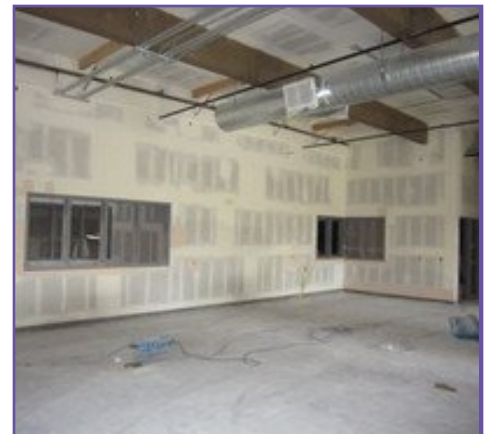
March —Sheetrock is placed on the walls.
